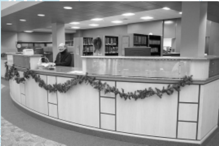
The installation of the Library's new Circulation Desk completed the year-long renovation
